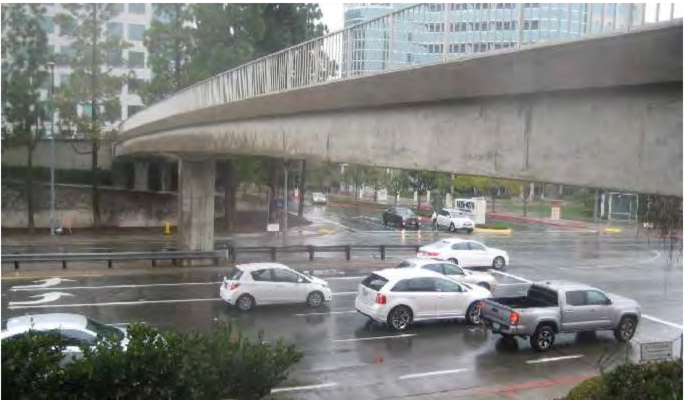
Figure 2: Photo facing west across Genesee Avenue near Executive Square, showing the current pedestrian bridge which remained at the time of the photo.
