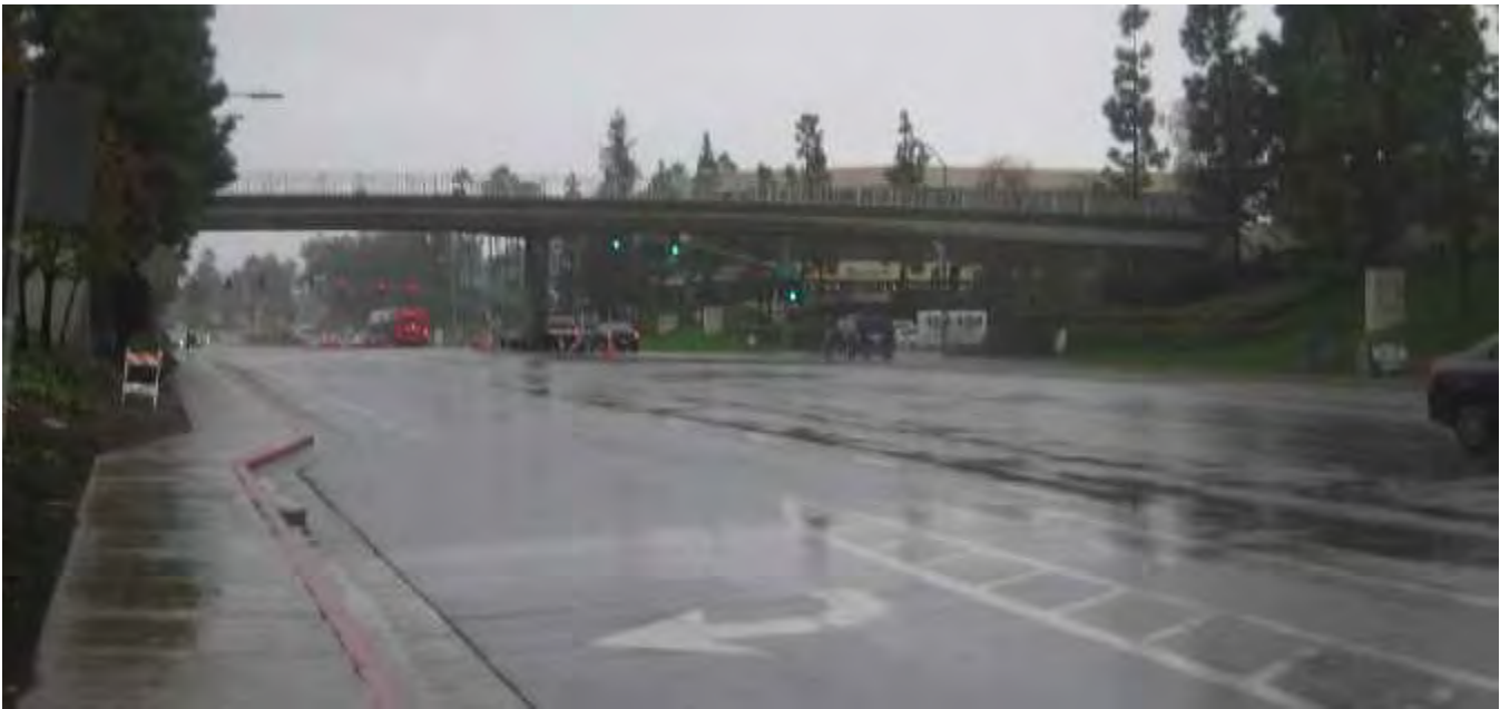
Figure 1: Photo facing north along Genesee Avenue toward the traffic signals at Executive Square and the current pedestrian bridge.
