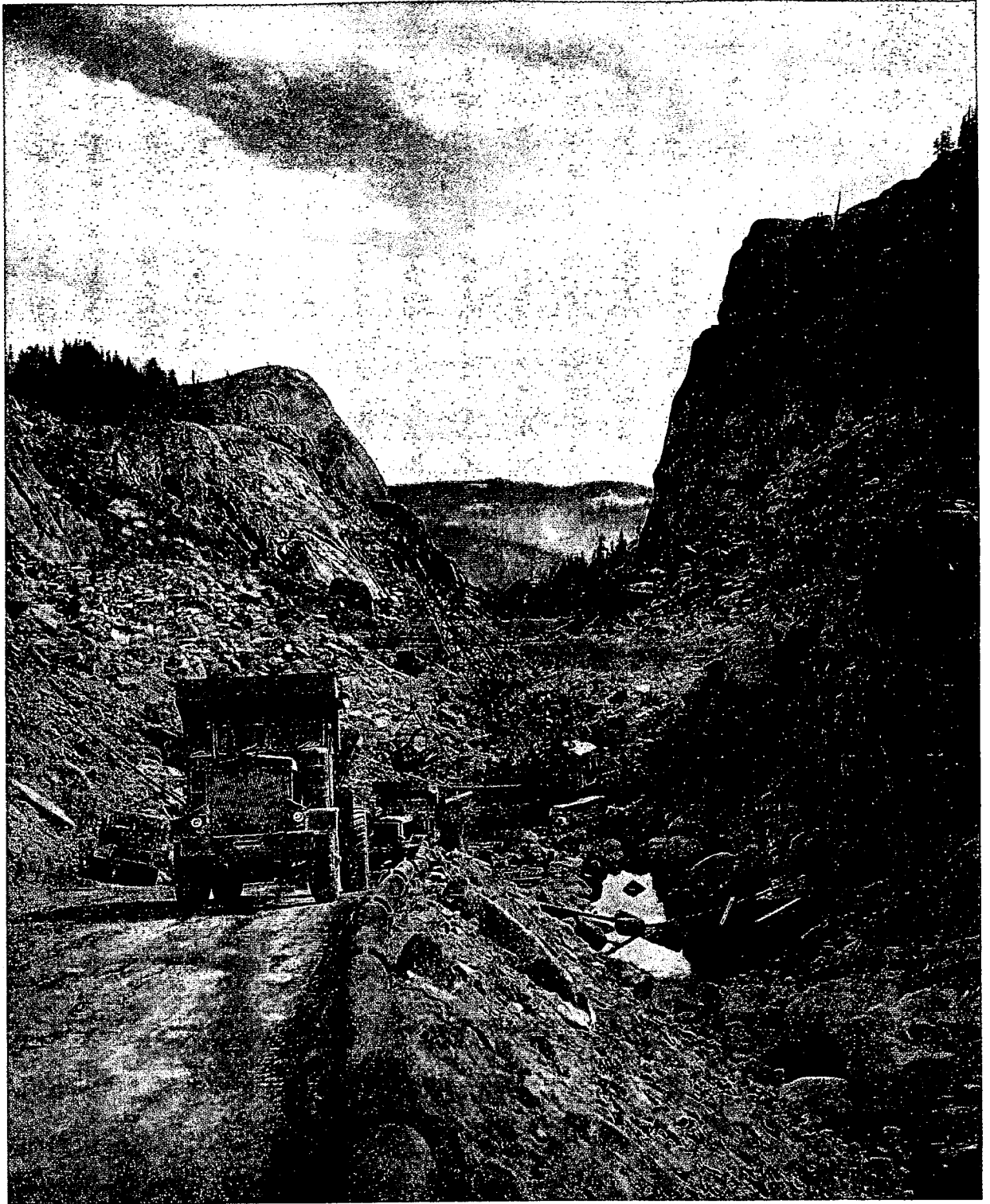
Foundation work in progress at the site of Courtright Dam, at an elevation of 8,000 feet, on the $80 million Kings River Development in the rugged High Sierra. Two dams, two new powerhouses, and the enlargement of existing facilities along the river will add 261,500 kilowatts of electric generating capacity to our system resources by the close of 1958.
