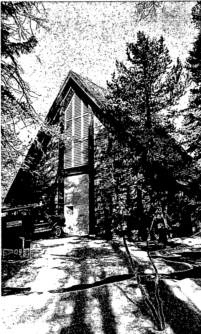
From the highway, this PG&E substation looks like a ski chalet. It serves a big, new, all-year recreational area in the Sierra.
