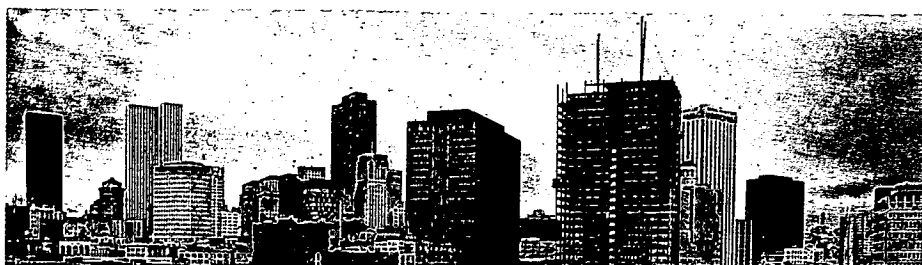
Steelwork for PG&E's new headquarters building rises toward San Francisco's changing skyline. A new low-rise structure links the 34-story tower and the present General Office building.
