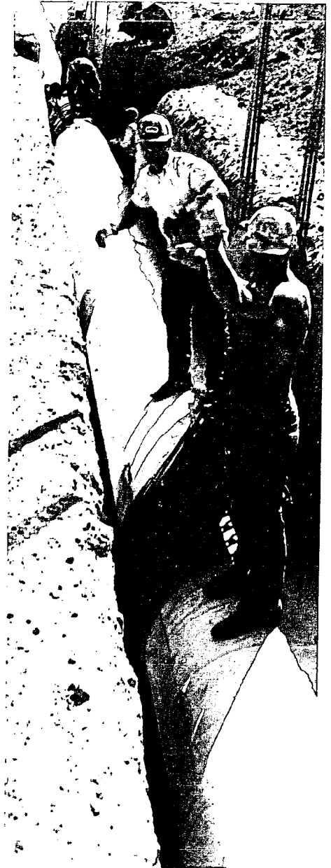
Sections of a 36-inch pipeline are lowered into a trench in Northern California as part of a program to expand the capacity of PG&E's Canadian gas line. This recently completed project enables PG&E to import 980 million cubic feet of gas a day from fields in Alberta, Canada.
