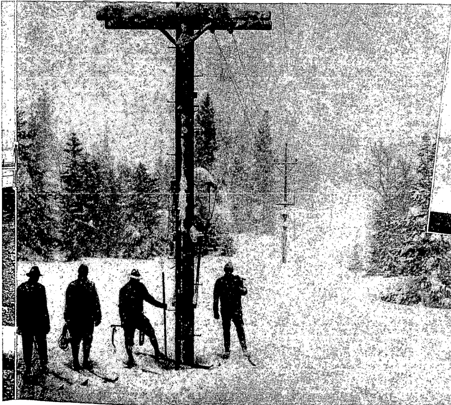
In winter snow, a ski crew patrols the Sierra-Spaulding transmission line.
