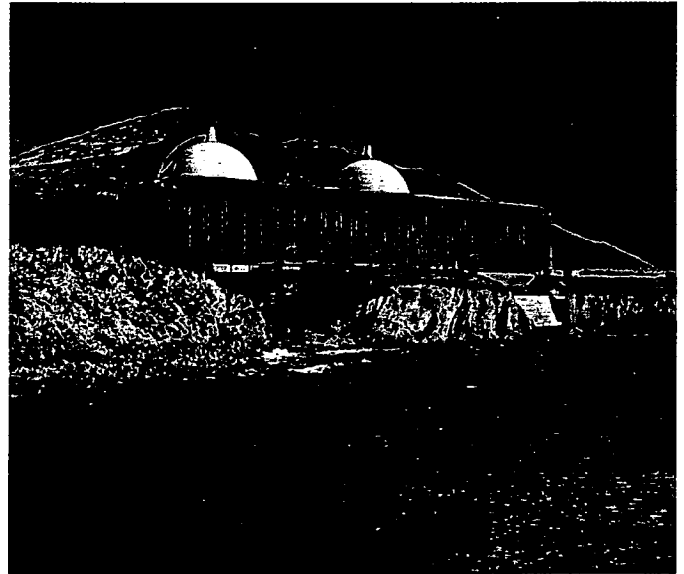
After 10 years of construction, PG&E's Diablo Canyon Nuclear Plant will produce power upon receipt of an operating license from the Nuclear Regulatory Commission.
