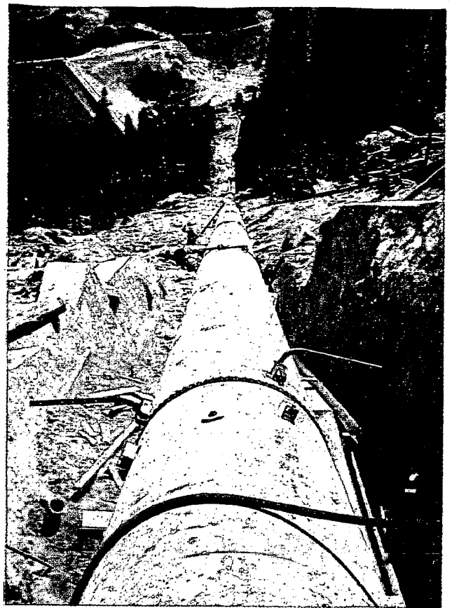
Through 4700 feet of steel penstock, water stored in the recently completed Bear River Reservoir is dropped to drive an added 29,000-kilowatt generator installed in Salt Springs Powerhouse on the Mokelumne River.
