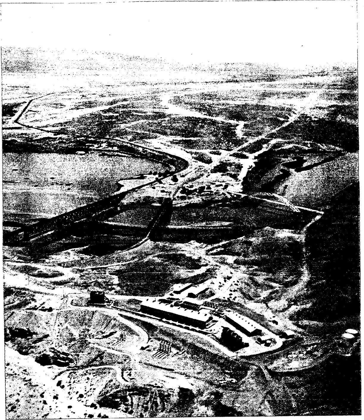
Topock Compressor Station. Located on the California-Arizona border, it is one of three compressor stations on the Company's 502-mile Topock-Miipitas gas transmission line, through which natural gas from out-of-state sources, principally from fields in Texas and New Mexico, is transported to our customers in Northern and Central California.
