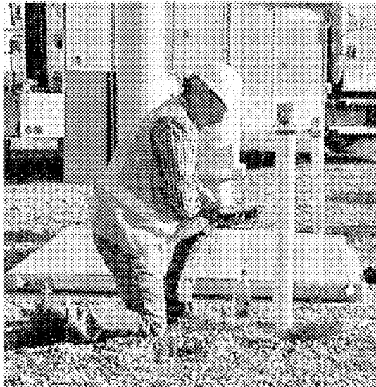
Technician Taking Pipe-to-Soil Potential Measurement
