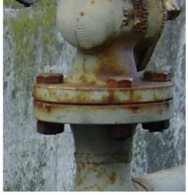
Atmospheric Corrosion compromises the integrity of the pipe, as it diminishes wall thickness of pipe. It consists of scaling, pitting, and/or blistering. Below are examples of atmospheric corrosion conditions that may require repairs:
