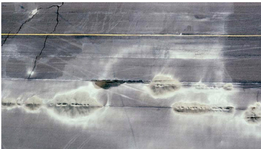
Figure 2. Sand volcanoes at the Oakland Airport runway, caused by liquefaction from the 1989 Loma Prieta earthquake.
