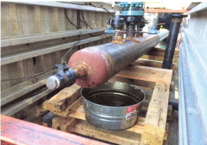
Test 022A-12 test 3 Loc. B testhead inside shoring box
