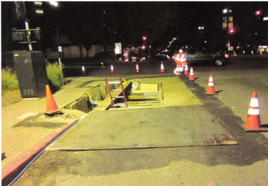
Test 022A-12 test 4 excavations on both sides of intersection
