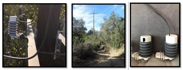
Figure 7 (a) Concealed lightning arrester (b) ductile iron pole (c) comparison of lightning arrestor models
