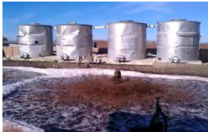
Aerators treating waste at work: PG&E's team of industrial energy efficiency experts continuously look for ways to further municipal wastewater facilities' energy efficiency opportunities.
