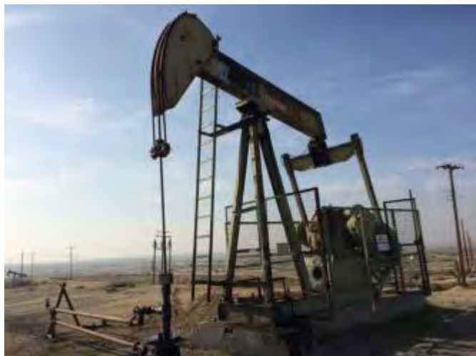
EnerNOC’s Energy Efficiency Services for Oil and Gas Production Program provides turnkey energy efficiency services that position oil and gas producers for high-level of energy savings and customer satisfaction.
