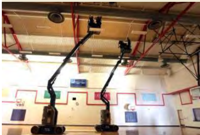
Direct Install Implementer Staples installs energy efficiency lighting inside the gym and activity center at a Bakersfield-area church.
