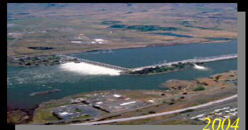
115kV Columbia River 2004
