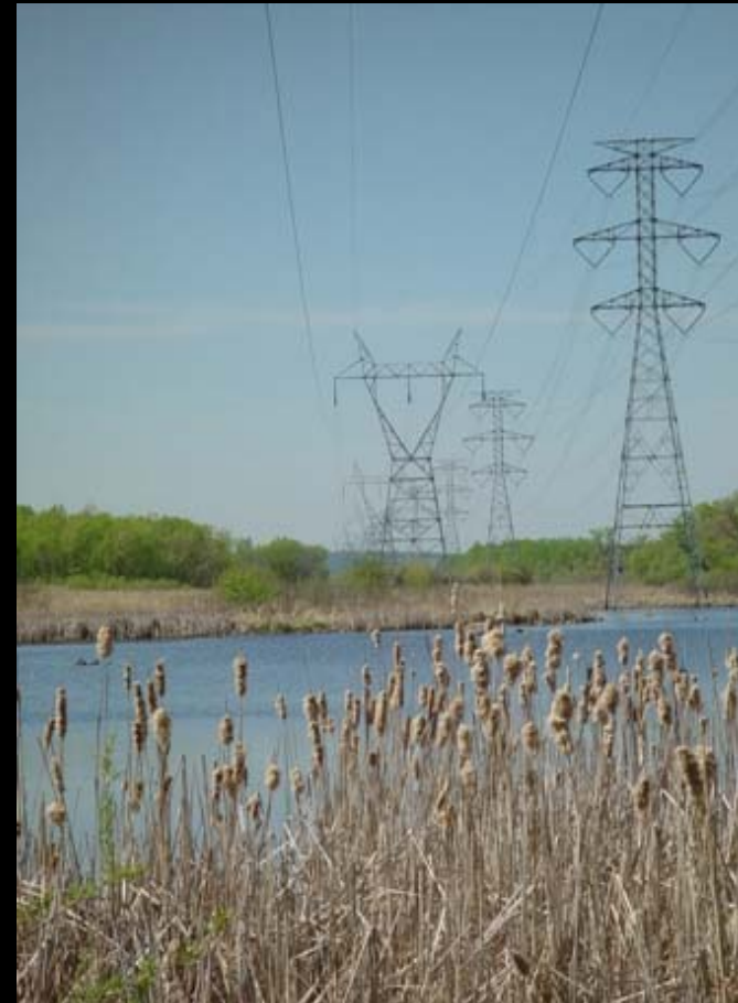
After Installing 3M ACCR (80% capacity increase)
