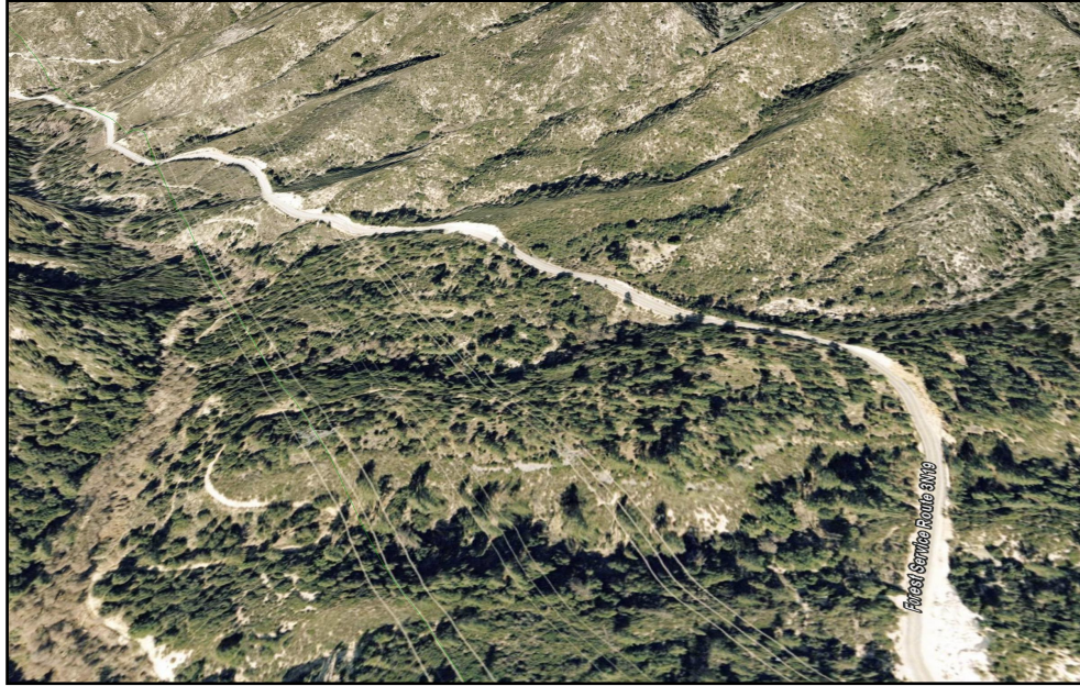
Photo 10: Aerial (oriented north) of potential shaft location where construction would switch from tunnel boring to cut/cover trench tunneling within Upper Big Tujunga Canyon Road (near S6 MP 16.0). Source: Google Earth.
