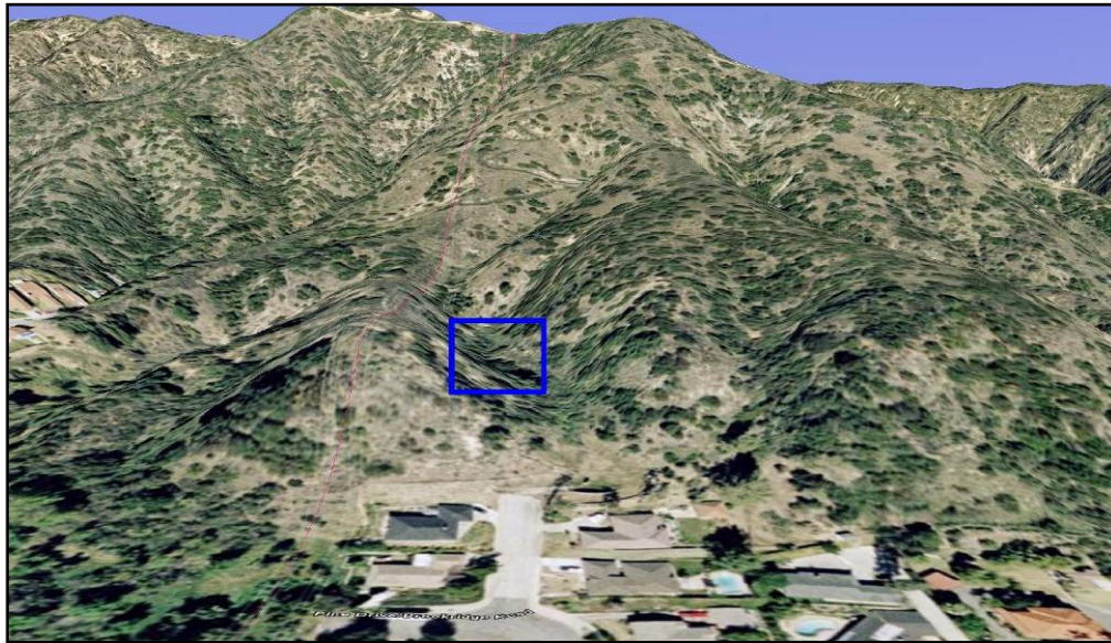
Photo 13: Aerial looking north at potential southern portal and transition station location in Duarte (near S7 MP 0.8). Source: Google Earth.
