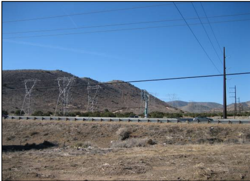
Photo 14: Looking northwest from Soledad Pass along Segment 5 (S5 MP 16.8) at Pleasant Valley.
