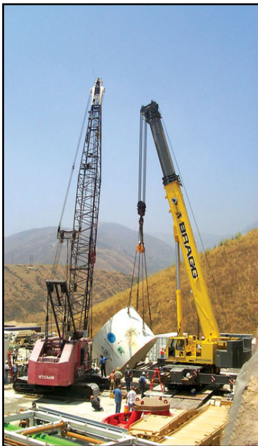
Photo 3 (Left): A 3900 Manitowoc Crane and a 300-ton Hydraulic Liebherr Crane were used to lift the front section of the tunnel boring machine.
