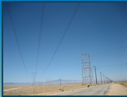
Segment 4 in NW Antelope Valley
