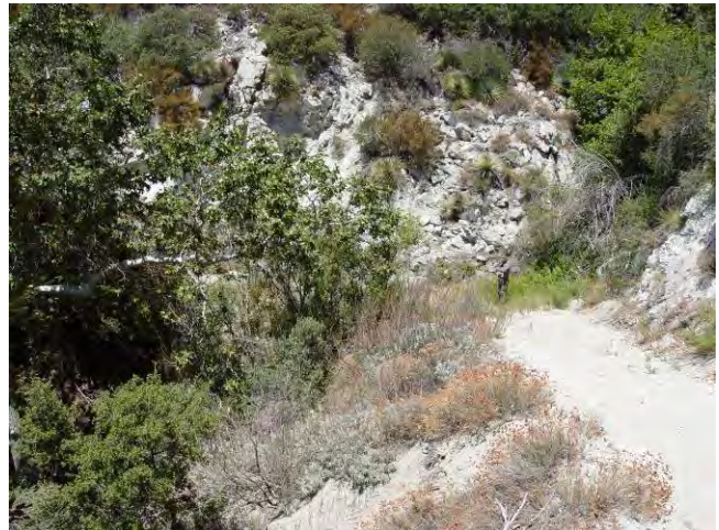
Buckwheat-lined road with steeply cut rock outcropping on the upslope.
