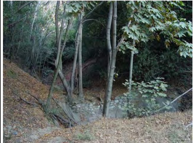
View of concrete and rip-rap drop structure just upstream from crossing.
