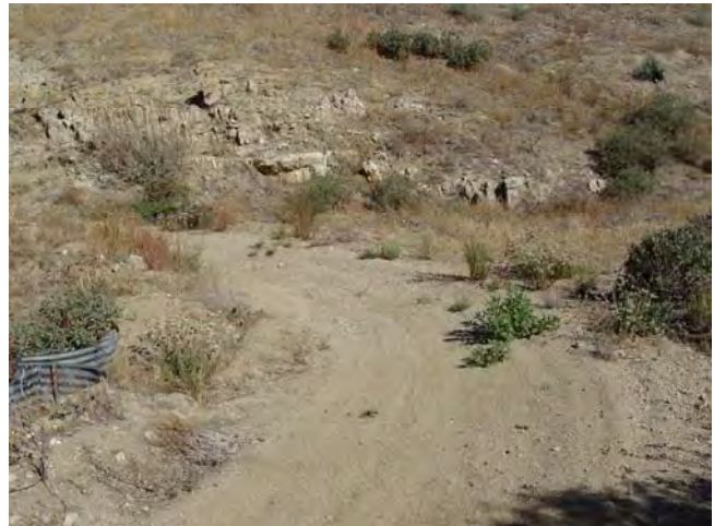
View along Edison Road (4N24.2) with drainage crossing in foreground of photo.
