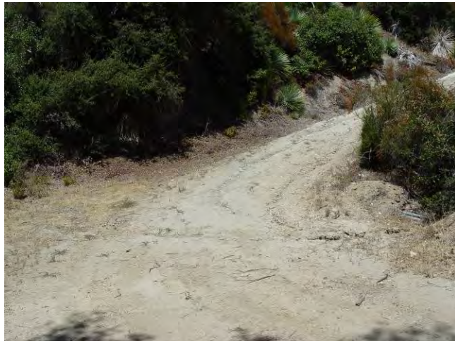
Barren pullout area on left with dense vegetation on upslope.
