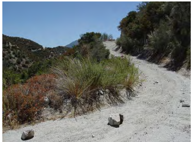
Road cut with steep upslope.
