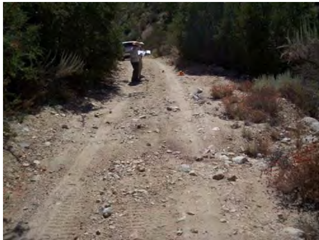
View along unnamed non-Forest System road. Note vegetation encroaching road.
