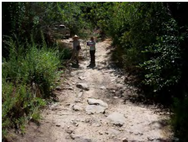
View along unnamed non-Forest System road. Note narrow road, dense canopy and riparian vegetation encroaching road.
