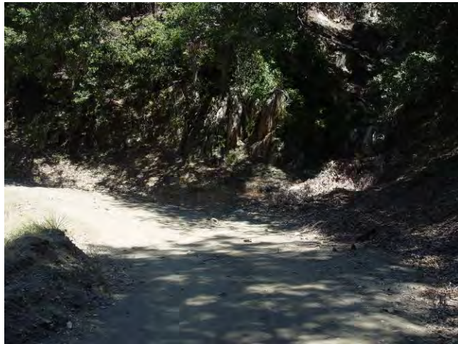
Road narrows around curve. Note steep upslope and dense canopy shading the road.
