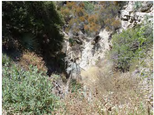
Drainage with steep, exposed rock wall and dense vegetation.
