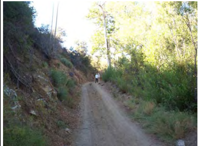
View along Lynx Gulch Road (4N18.2) just north of the crossing. Note narrow width of road, steep embankment on one side of the road and dense vegetation along the other side.
