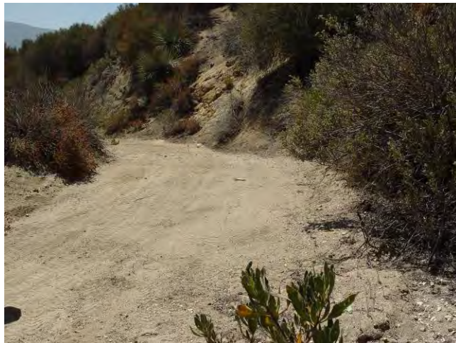
Note wide road width at this location.
