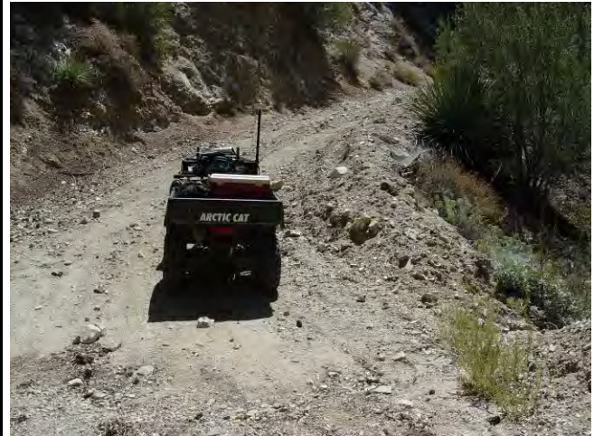
Note loose rock debris on road.
