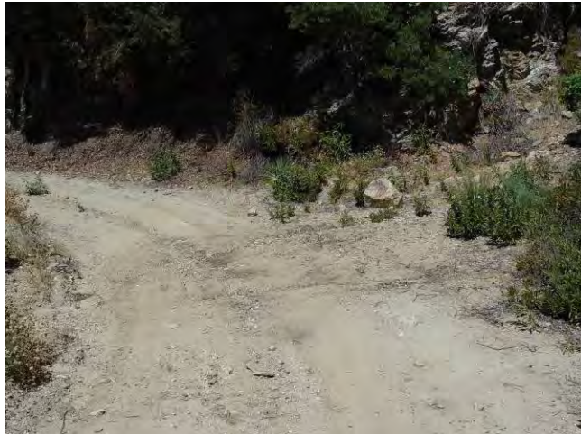
Ephemeral drainage comes down hillside and crosses road here.
