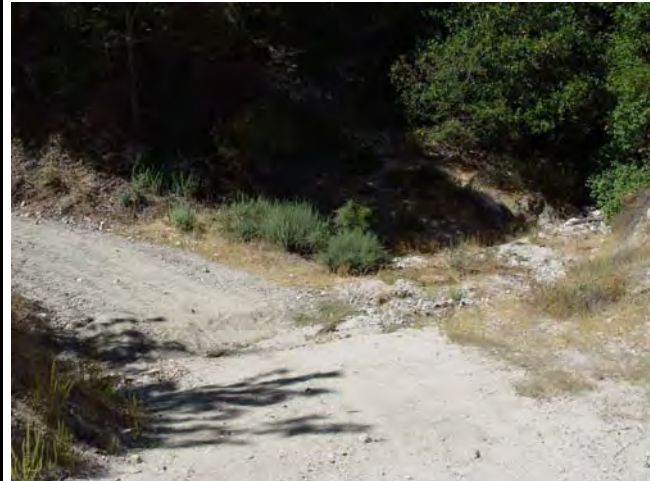
View of tributary drainage crossing along Shortcut Edison Road (2N23). Note annual grasses along road edges.
