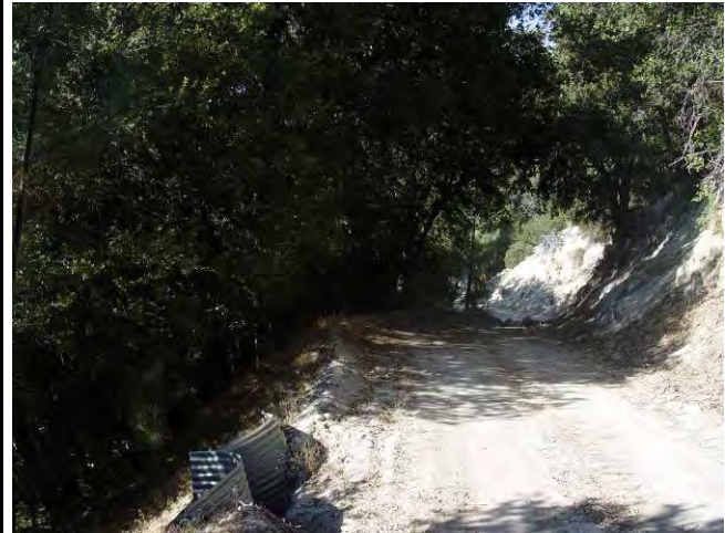
Note McCarthy drain and steep upslope and down slope. Mature trees form a canopy over the road.
