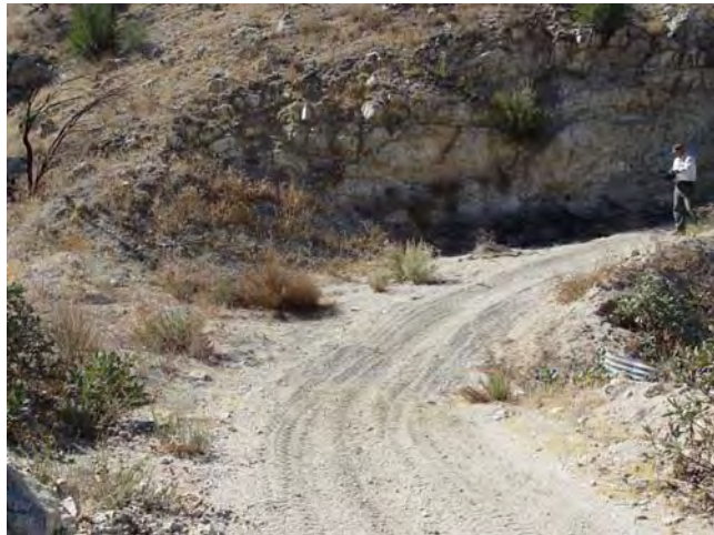
View along Edison Road (4N24.2). Note steep exposed bedrock wall along roadside.
