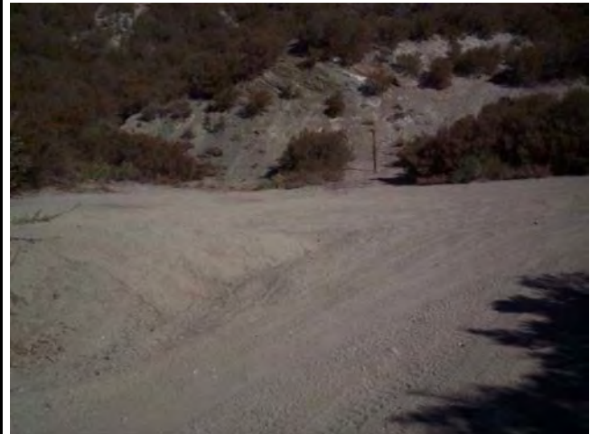
View along Monte Cristo Creek Road (3N23) just north of crossing. Note barren area at turnout.
