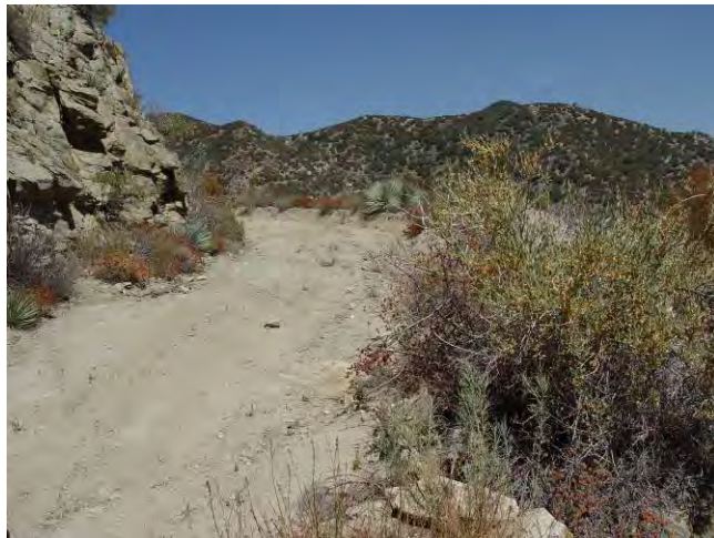
Steep bedrock wall on the upslope.
