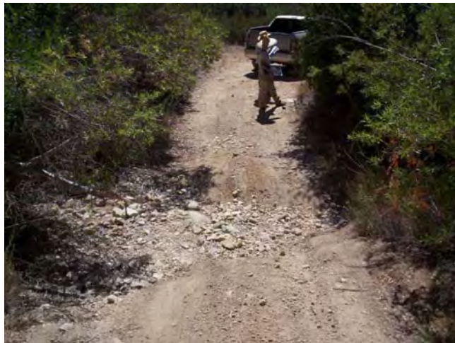
View along unnamed non-Forest System road. Stream cuts deeply into road here. Note dense riparian vegetation along narrow road.
