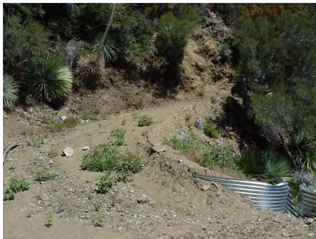
Note steep upslope and drop off from road. Vegetation is growing within roadbed.
