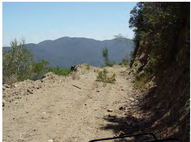
Note steep upslope and drop off from road.
