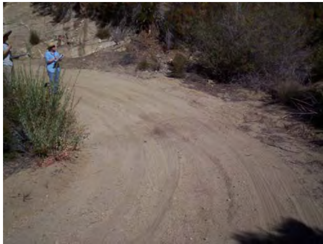
View along Powerline Road (3N20). Note vegetation along roadsides.
