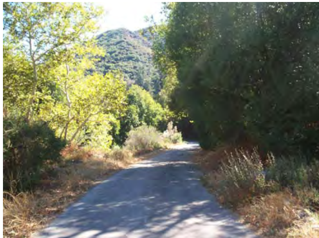
View along 2N25.1. CMP is present beneath road crossing at this location.
