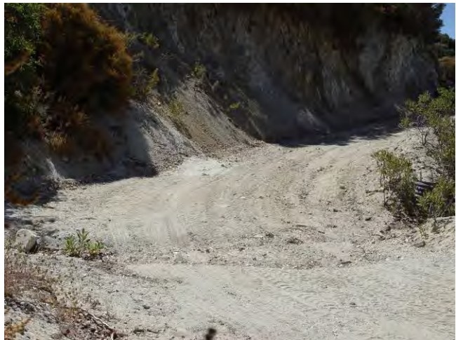
Road cut with steep upslope. Scour line from flows can be seen crossing the road in the foreground.
