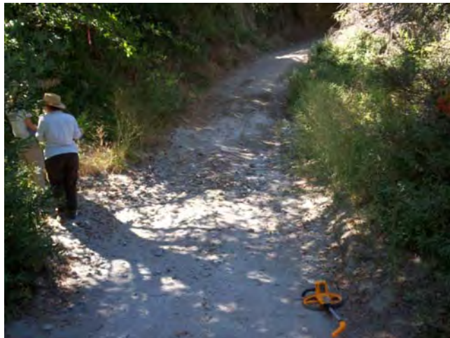
View along Monte Cristo Creek Road (3N23). Note very narrow road width with encroaching vegetation.
