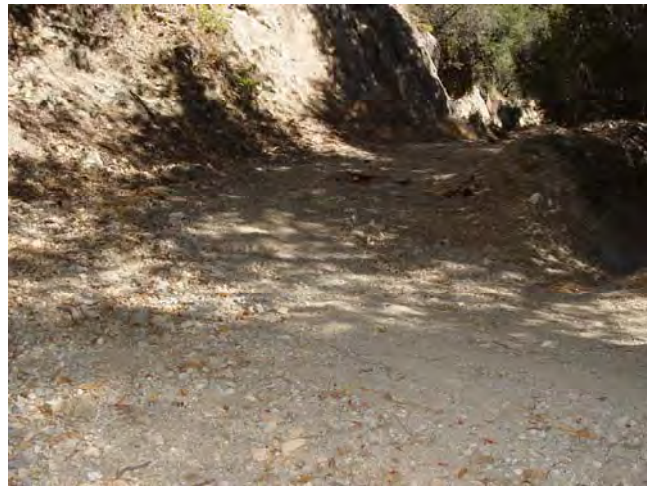
View along Shortcut Edison Road (2N23) at crossing location.
