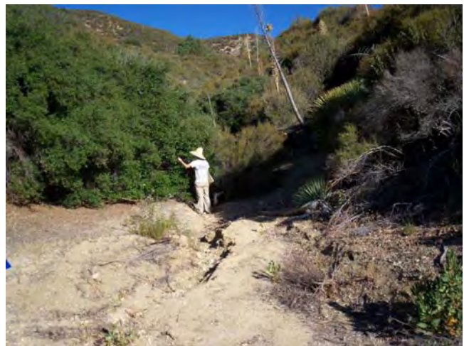
View from road towards upstream portion of drainage. Note no riparian vegetation.
