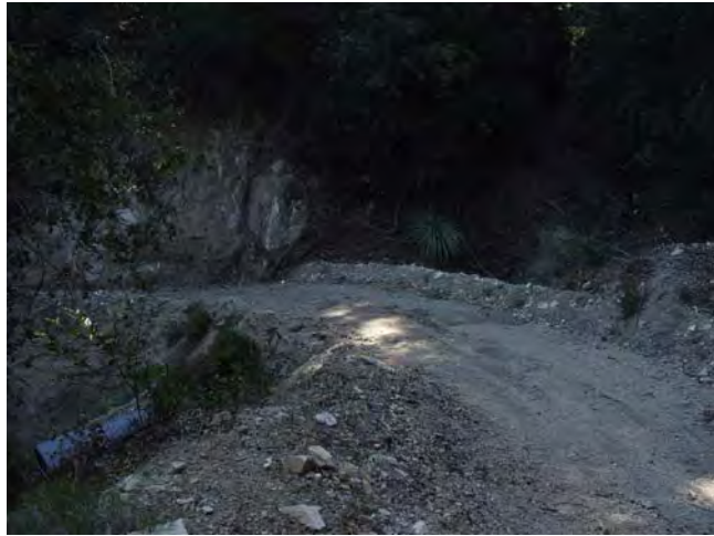
View along unnamed road. Note CMP at crossing.
