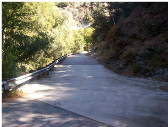
View along 2N25.1 with guard rail along northern edge of road.
