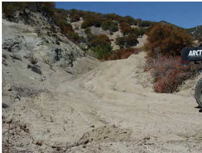
Exposed areas of clay and bedrock with chaparral surrounding.
