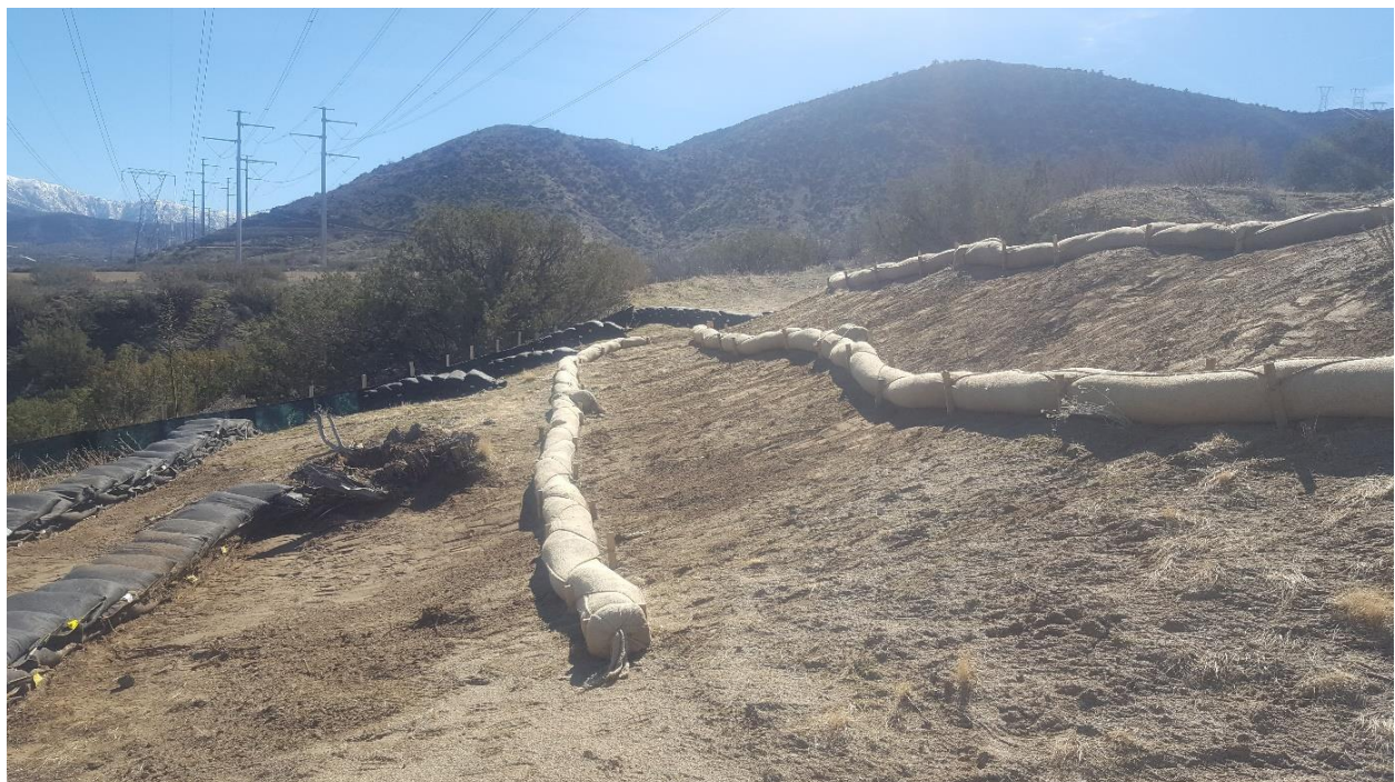
Figure 6: Tower 6 after BMP maintenance, Segment 6. Photo courtesy of SCE.
