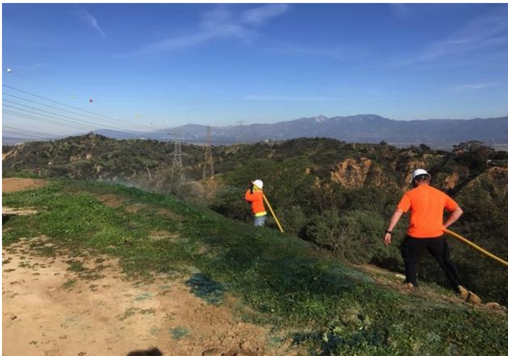
Figure 2: Hydroseeding at Segment 8 Restoration Site 023. Photo courtesy of SCE.
