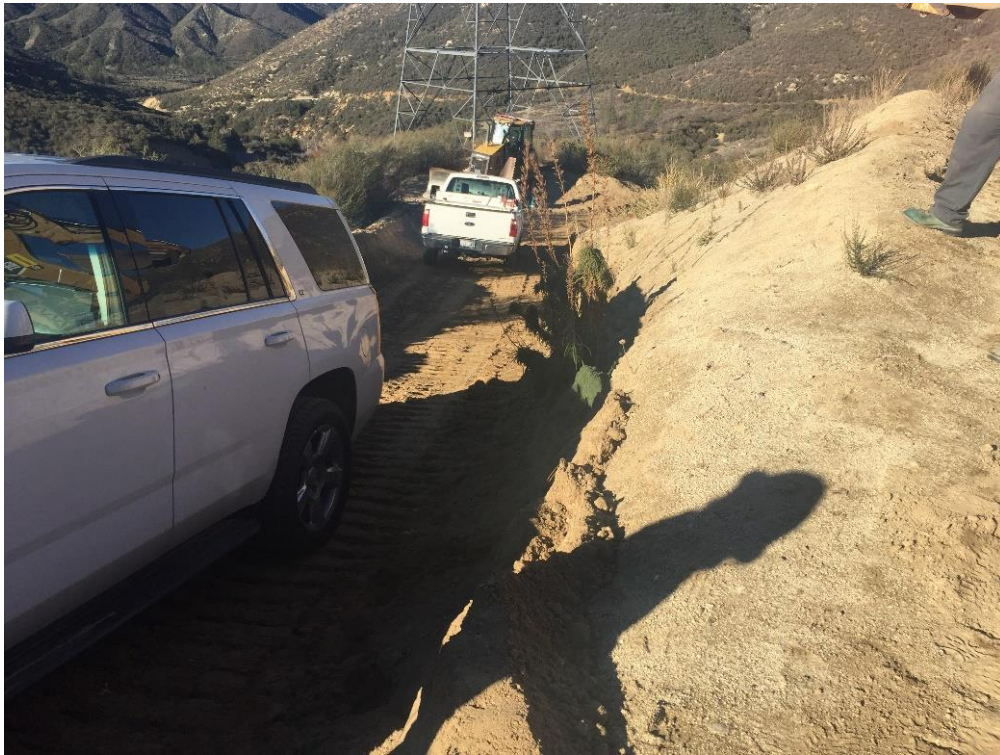
Figure 1: Grading crews restoring access road near Tower 59 “give back area,” Segment 6.
