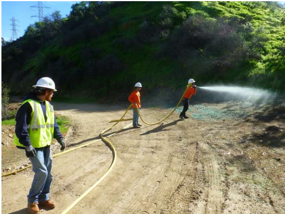
Figure 4: Hydroseeding at Restoration Site R035, Segment 8 Phase 4. Photo courtesy of SCE.
