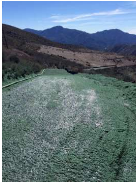
Figure 2: Rabbit Peak HAY entrance after hydroseeding. Photo courtesy of SCE.
