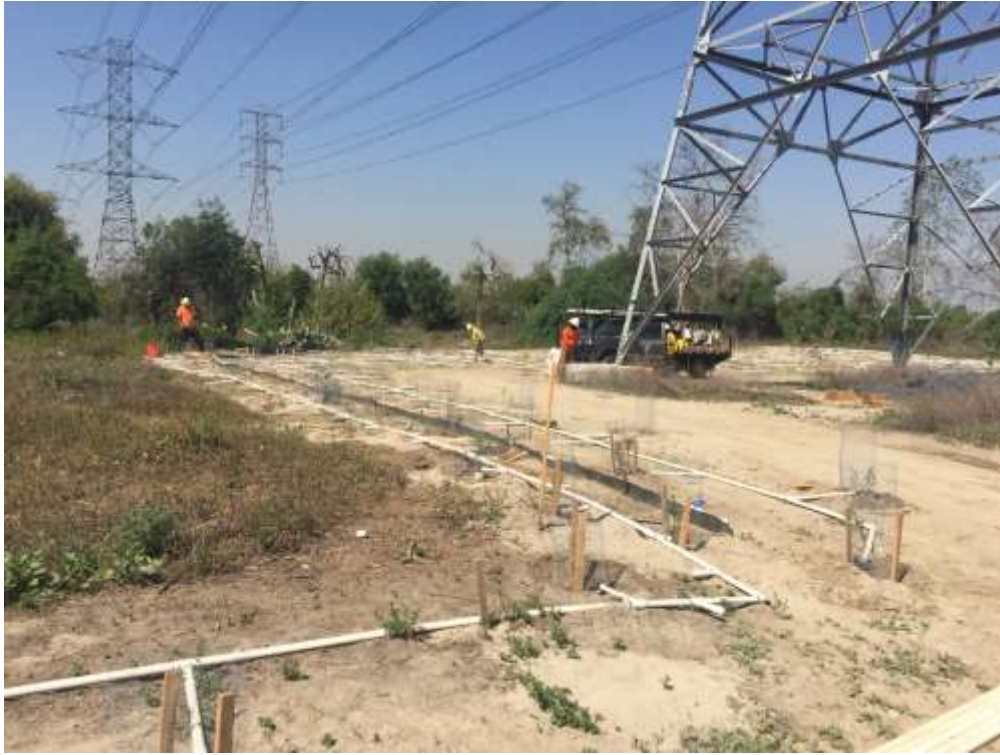
Figure 5: Container plant installation at Restoration Site R0006, Whittier Narrows, Segment 8.
