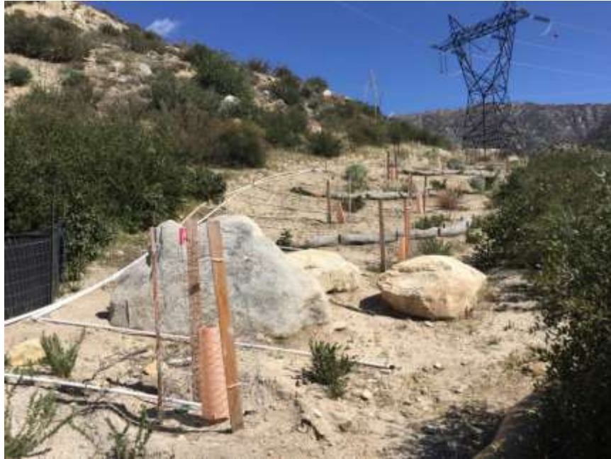
Figure 1: Pull Site 28/29 after BMP maintenance, Segment 6.
