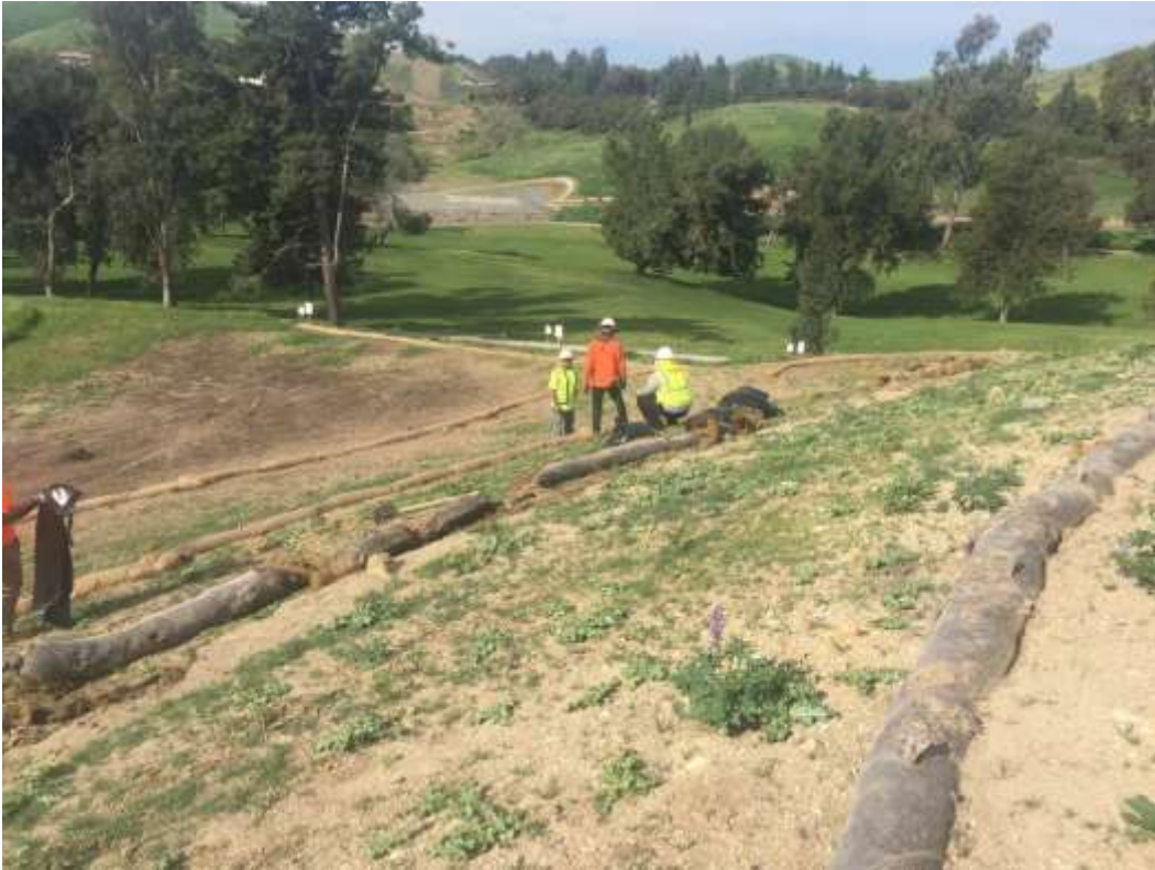
Figure 7: BMP maintenance and repair near Vault Cluster #3, Segment 8 Underground.
