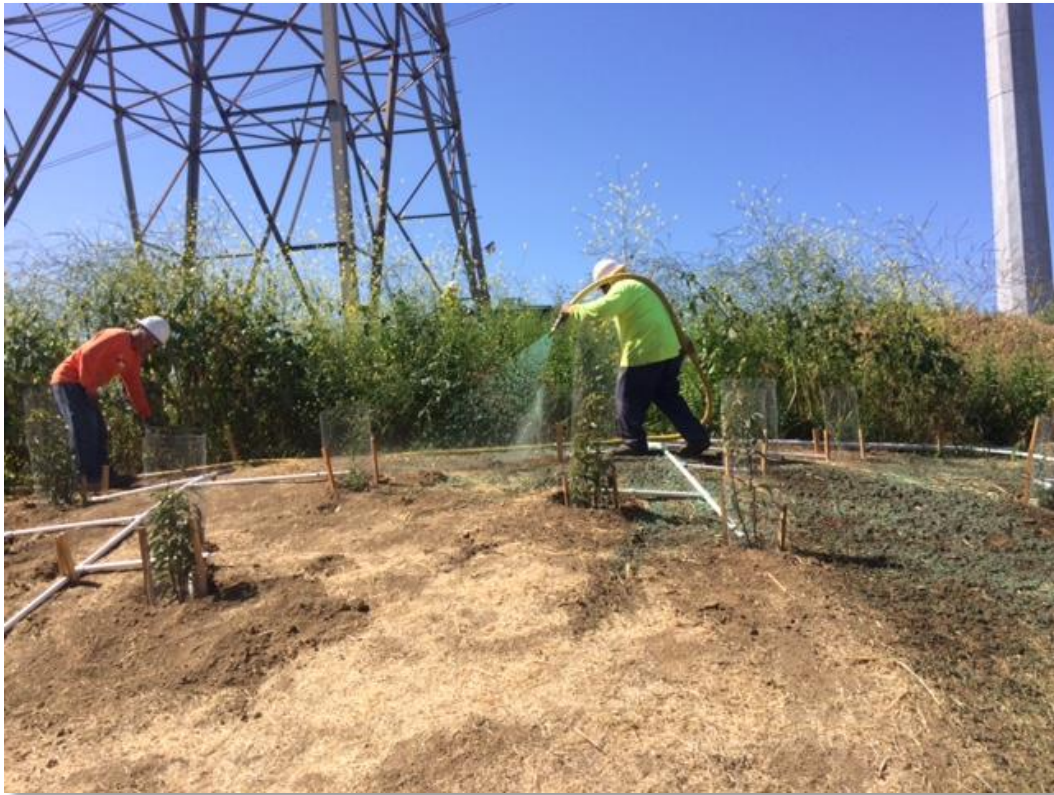
Figure 3: Segment 8 restoration Site R27 during hydroseeding activities. Photo courtesy of SCE.
