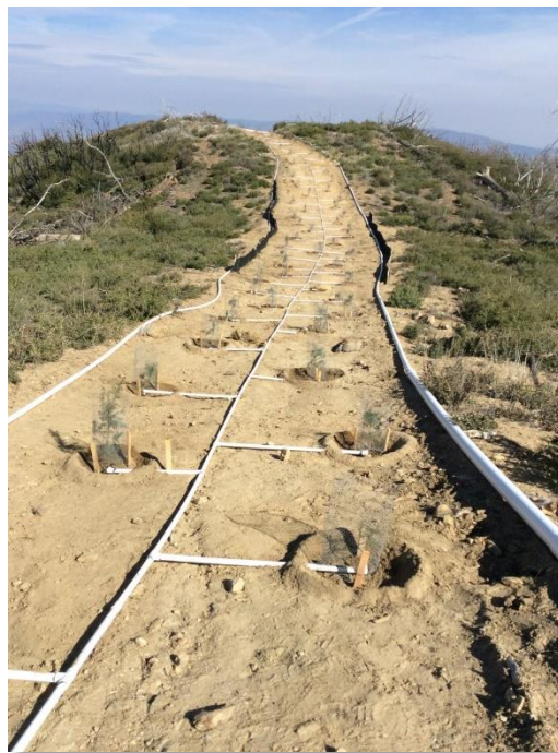
Figure 2: Segment 11 restoration site R47 after container plants were installed. Photo courtesy of SCE.
