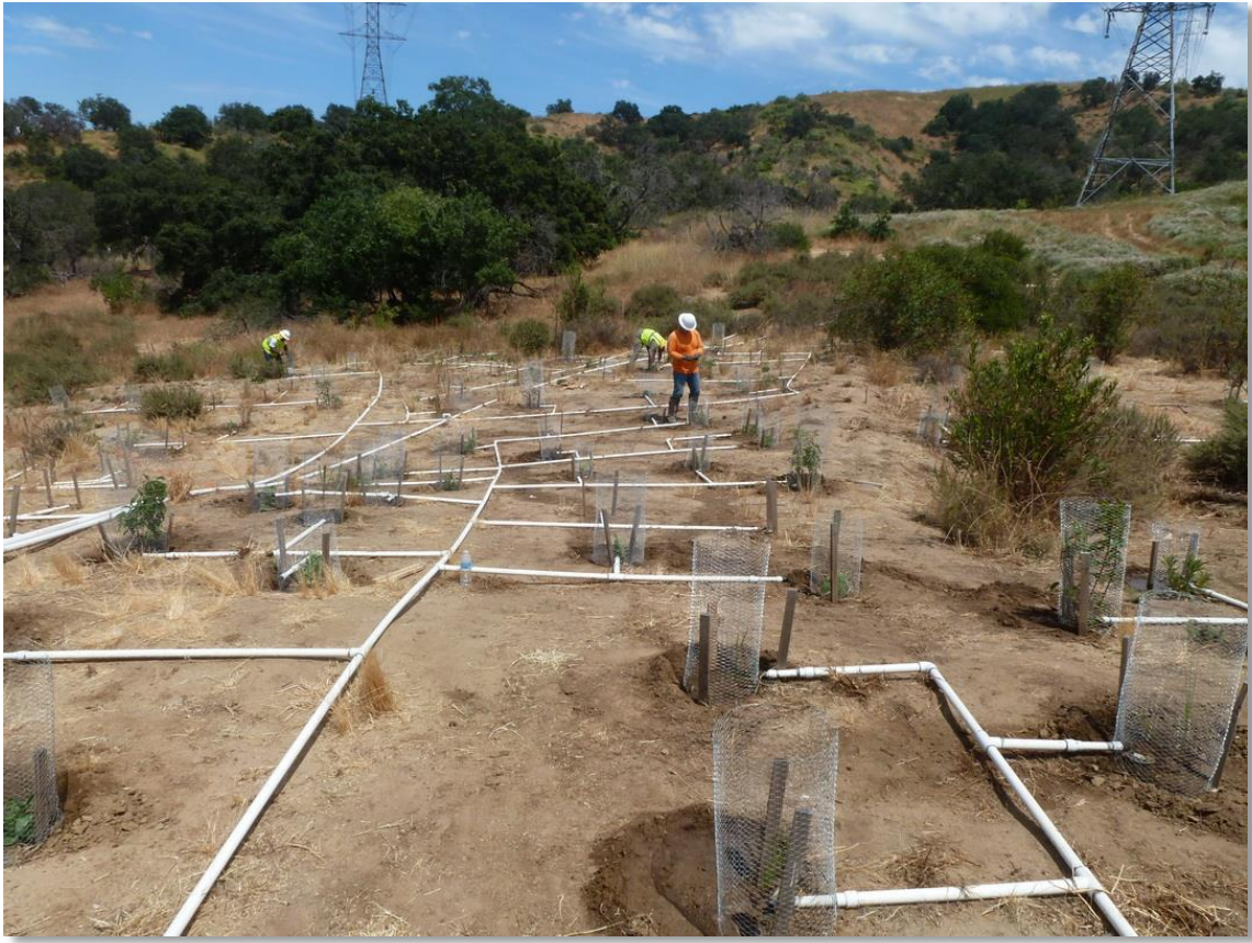
Figure 1: Container plant installation at Segment 8 restoration site R78. Photo courtesy of SCE.
