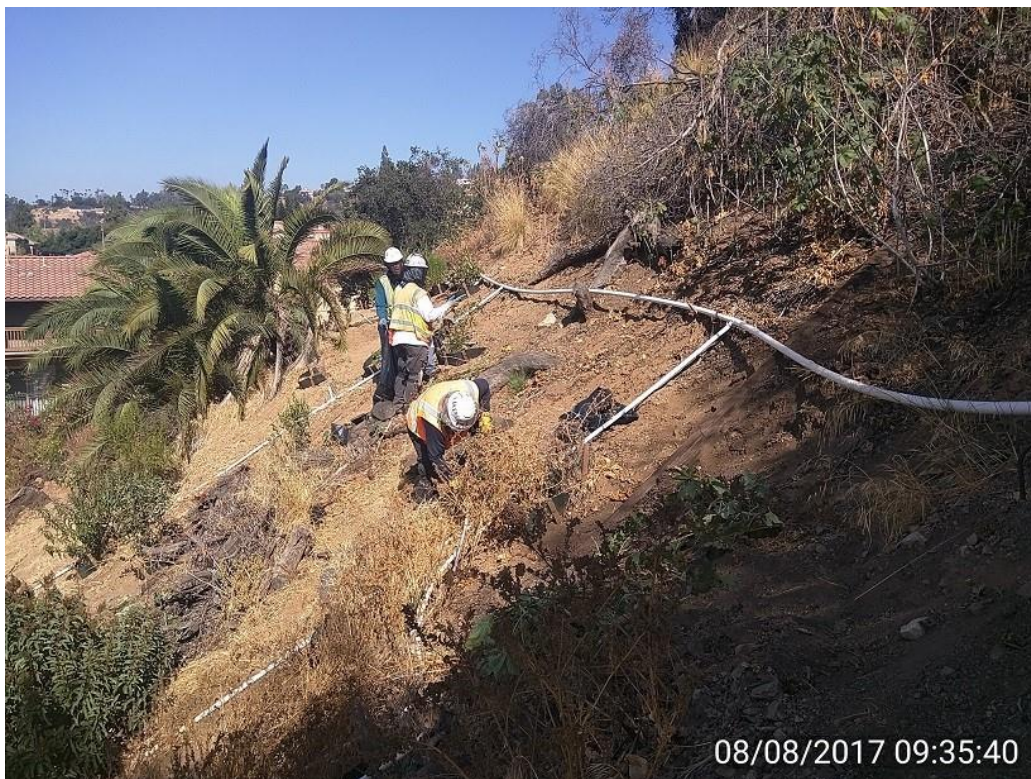
Figure 2: Weed abatement at Restoration Site 03, Segment 7. Photo courtesy of SCE.
