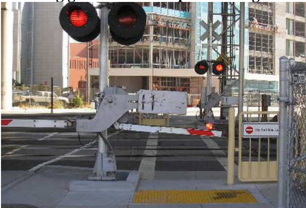
Figure 6. Example of an emergency exit swing gate used with a pedestrian gate
