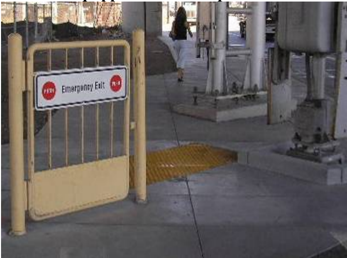
Figure 10. Emergency exit swing gate equipped with a kickplate
