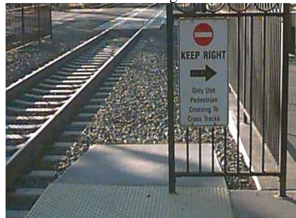
Figure 39. Ballasted area between platform and crossing
