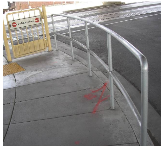
Figure 45: Channelization using steel tubular fence
