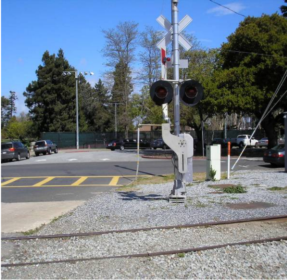
Figure 47. Pedestrian automatic gate without channelization
