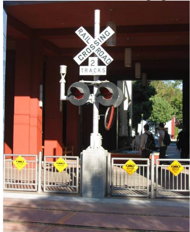
Figure 3: Example of entry/exit swing gate with LOOK BOTH WAYS signage
