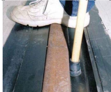
Figure 26. Inserts reduce gap depth
