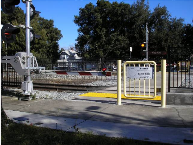
Figure 5. Example of emergency exit swing gate with Do Not Use Gate signage for pedestrians approaching the crossing
