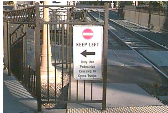
Figure 38. Railroad worker's ramp near crossing
