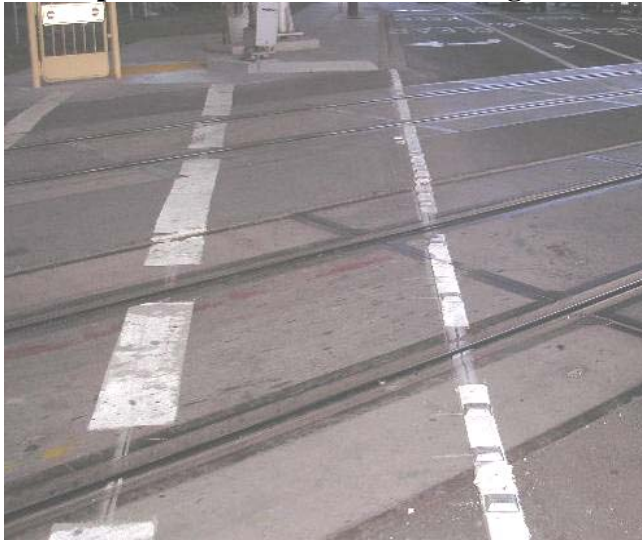
Figure 36. Example of white reflective raised-pavement-markers with an edge
