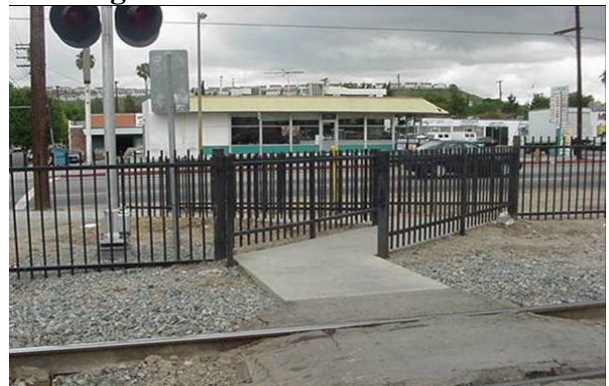
Figure 51: Z-Gate with flasher unit
