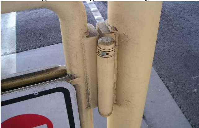
Figure 8. Hinge welded to post
