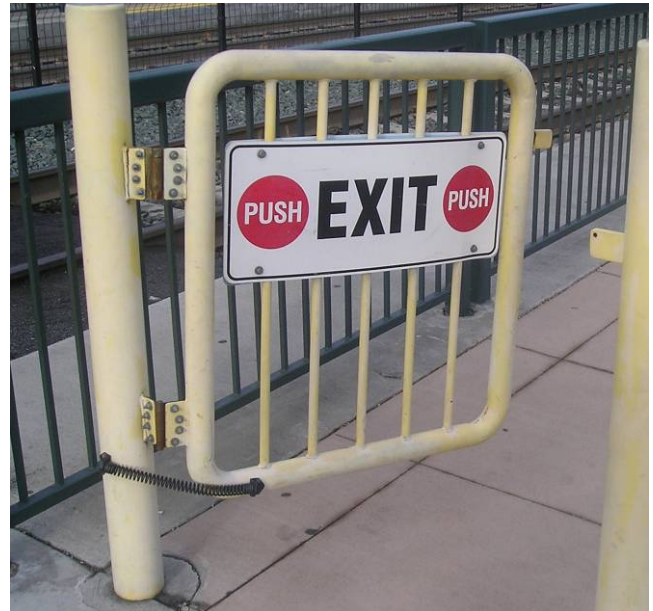
Figure 7. Example of emergency exit swing gate with Exit signage as viewed from the track side
