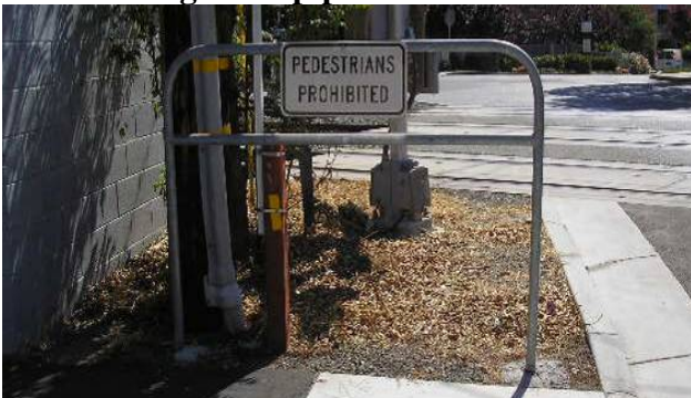
Figure 29. PEDESTRIANS PROHIBITED sign and pipe-rail barrier
