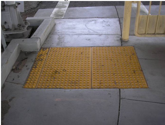
Figure 12. Detectable warning surface at edge of curb
