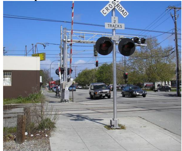
Figure 48. Flashing light signals for pedestrians in off-quadrant
