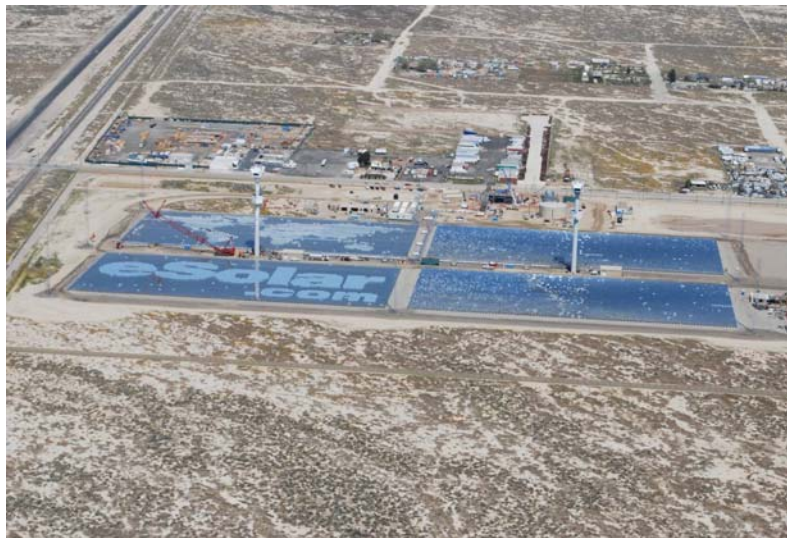
Aerial photograph of the Sierra SunTower site.
